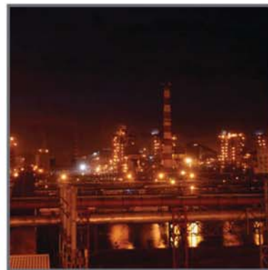
JINDAL POWER STATION
